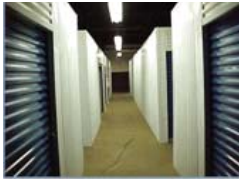
BDI Warehouse, Detroit MI
